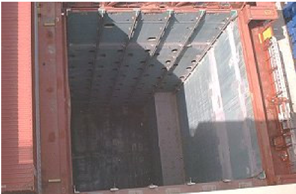
Figure 2.4) Cargo hold with cell guides. Source: www.containerhandbuch.de (acc: 2004-06-30)
